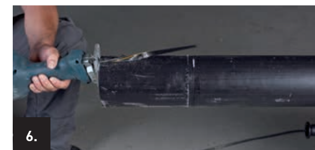
Cut the jacket down to the PUR insulation layer using a standard tiger saw or foxtail equipped with a plastic saw blade.
