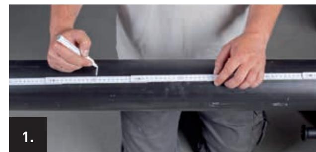
Measure the pipe length and mark it on the casing pipe.
