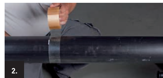
Mark the cutting line on the pipe circumference with adhesive tape.
