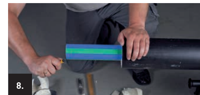
Clean the stripped carrier pipe and deburr the pipe end both internally and externally.
