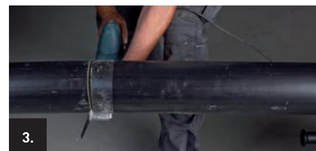
Cut the pipe along the cutting line using a standard tiger saw or fox-tail equipped with a plastic saw blade.
