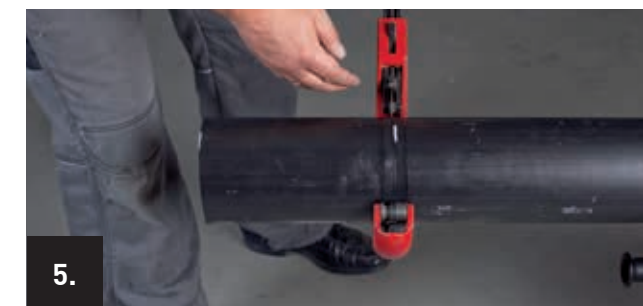
Cut through the entire circumference of the casing pipe with a pipe cutter up to the PUR insulation layer.
