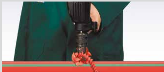
Drilling through the pipe wall
