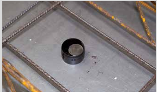
Base part of sprinkler outlet Art. no. 3090000001 for visible sprinklers. Attachment by magnet.
