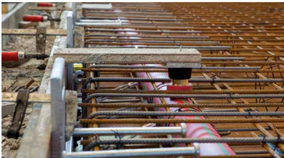
Prefabrication concrete wall
