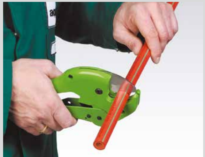
Cutting of the pipe
