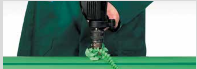
Drilling through the pipe wall
