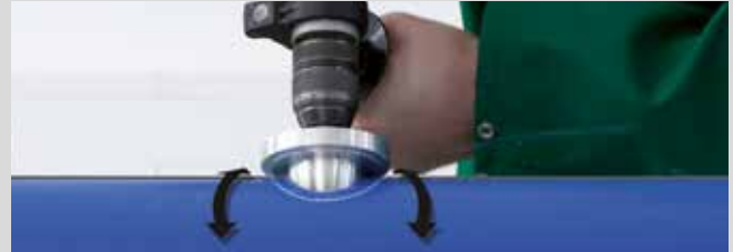
Removal of the oxygen barrier layer from the aquatherm blue OT-pipe
