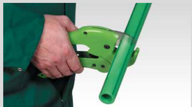
Cutting of the pipe
