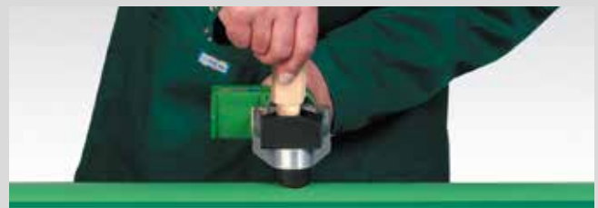
The welding tool is inserted into the pipe wall ...
