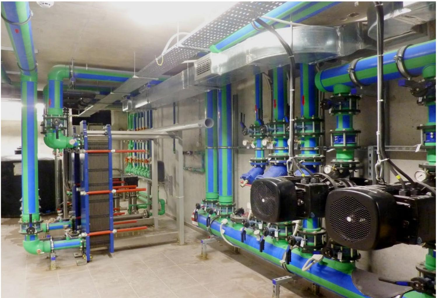
The entire piping of the heating and cooling circuits in the building including the connection to the geothermal system and the heat exchangers was realized with products from aquatherm: aquatherm blue pipe and aquatherm green pipe.
