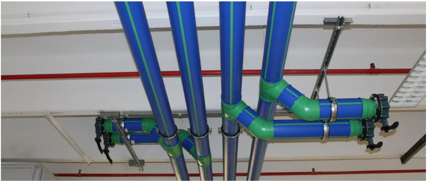
*“With our old system made of steel we had to struggle with incrustation, which resulted in increased energy consumption and thus additional costs”, says Egetenmeier. “The material polypropylene offered the perfect solution for this”.*
